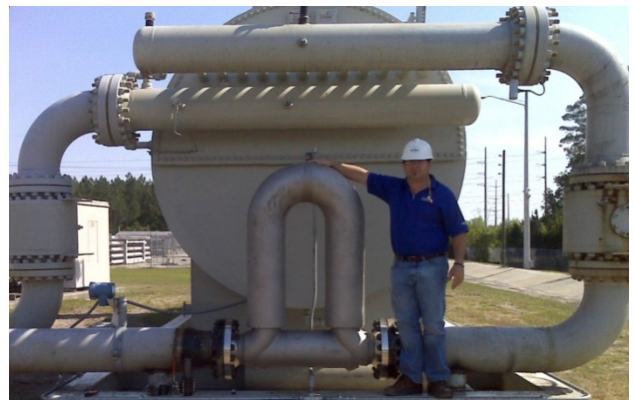
200mm (8") Coriolis meter installed in 250mm (12") line
