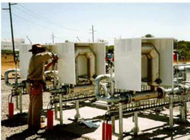
“After” installation since 1996, with two operating and one “hot spare” meter for 80:1 turndown.
