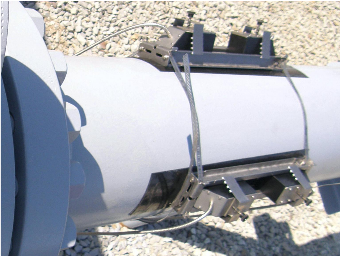
Figure III. Transducers mounted on pipe in reflect mode.
