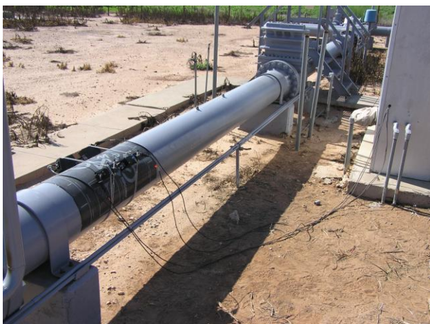
Figure IV. Clamp-on Compared to Orifice Meter
