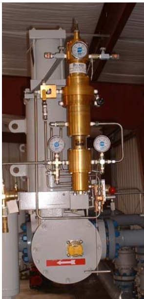
Ball Valve Regulator with Spring Return Actuator and PID Pilot Controls
