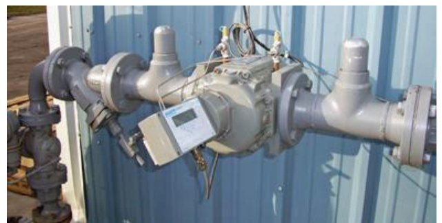
Integral Volume Corrector with Differential Pressure Capability
